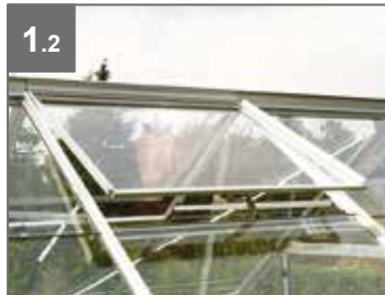
1.2 Window Exterior view
